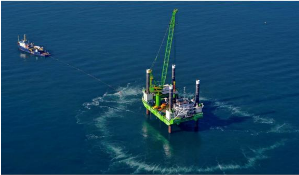
Figure 3. Big Bubble curtain around a construction site ( link ).
